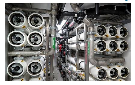
MPW'S REVERSE OSMOSIS SYSTEM LEADS TO DUAL COST SAVINGS AT OIL REFINERY Not satisfied with the variable cost of city water and the additional sewer charge associated with disposal of wastewater, managers at a Michigan oil refinery sought to restructure its water system by incorporating reverse osmosis (RO) technology. Plant personnel determined that reusing process wastewater would maximize efficiency and minimize expenses.
