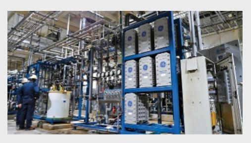
contacted MPW Industrial Services for the purchase and installation of the newest EDI technology through MPW's Products Direct arm (https://sales.mpwservices. com/), an E-Cell MK-3 from General Electric, now Suez. Plant management said it wanted to switch to the new technology during an upcoming five-day outage.
