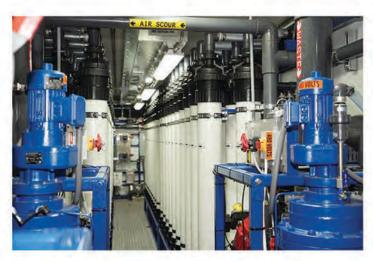
MPW's mobile ultrafiltration system can treat up to 1 million gallons of wastewater per day for as long as 8 months.
