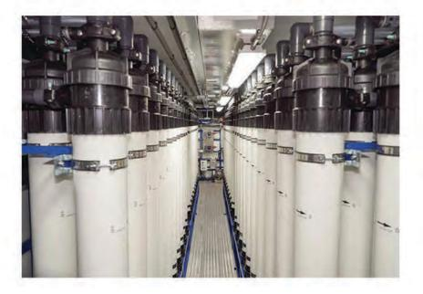
MPW's system consists of two independent racks, each capable of processing 400 gallons per minute. Redundant racks enable one to be cleaned while the other processes wastewater.
