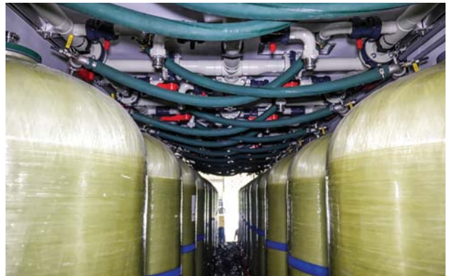
The demineralization trailers feature a capacity of 10 million grains.
