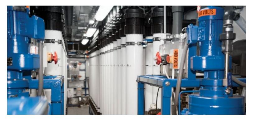
When a power plant required additional high-purity boiler feedwater for its startup following a major refurbishment, management requested temporary vendor support, which is a bread-and-butter assignment for the mobile water purification industry.
