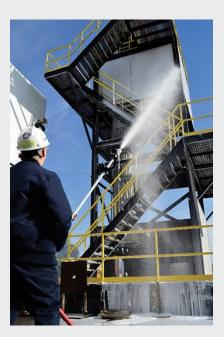
to natural gas, they needed to eliminate 30 years of coal ash and dust from the plant before the transition could take place. The company enlisted MPW and its foam cleaning method to ensure the highest standards of safety and efficiency were being met, but three decades of accumulated filth would not disappear easily.
