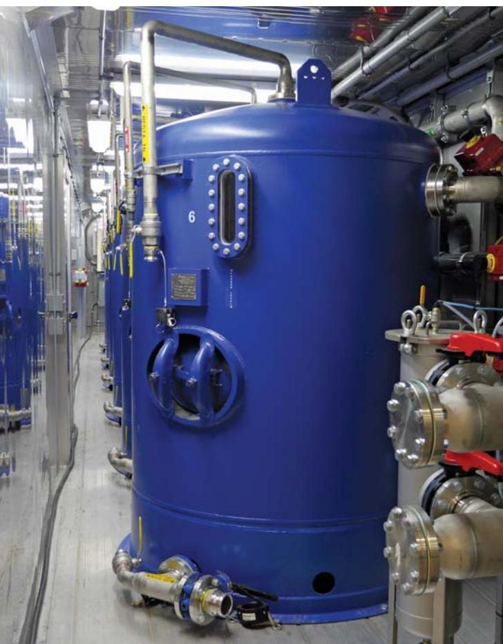
The trailer-mounted filtration system treated a portion of the mill's water, which then was blended back into water from existing filtration solutions.
